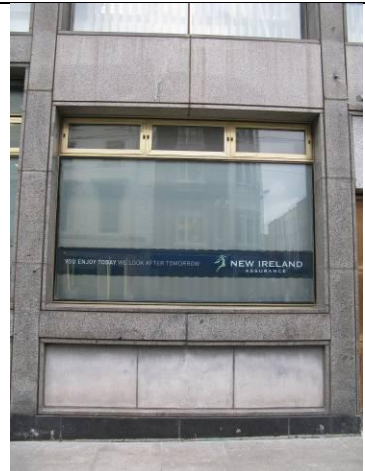
Ground floor bronze casement, granite framed with limestone apron
