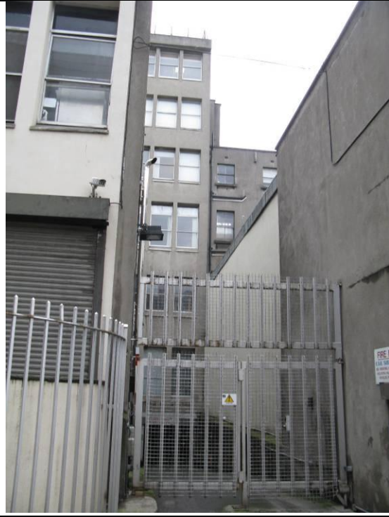
Access to underground area of Building C from Dawson Lane
