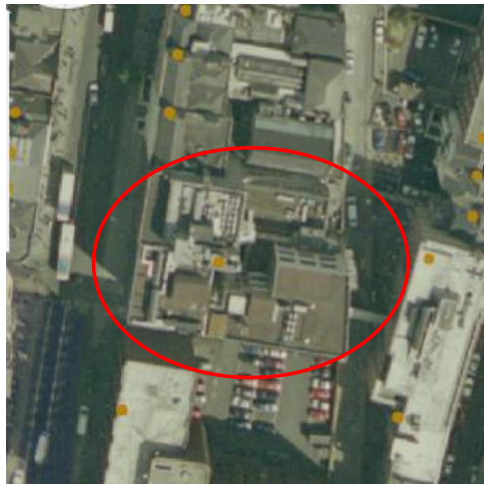
Aerial view of 9-12 Dawson Street & Dawson Lane, encircled in red
