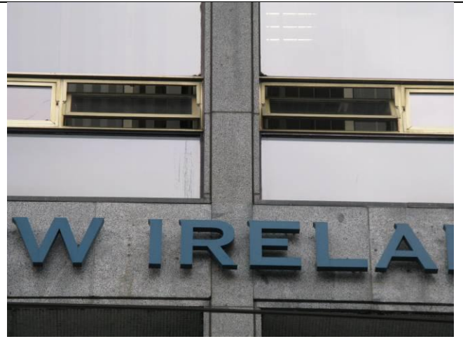
Central pivot bronze casement windows in use
