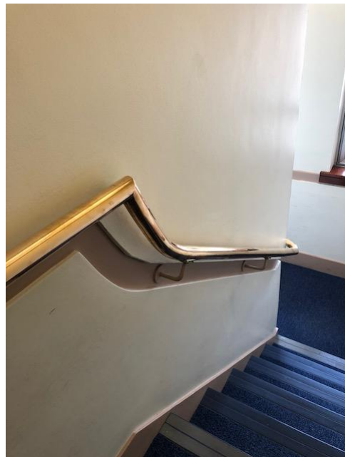
Original internal handrail along the original stair-core of Building A
