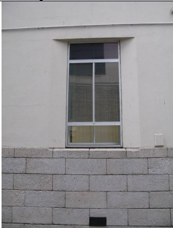
Splayed reveals and chamfered granite cill with Ashlar granite plinth
