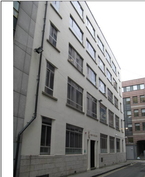
Building A: entrance on Dawson Lane
