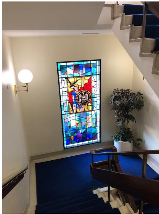
All original stained glass to Building B still exists in situ. Terrazzo staircase is fully intact from basement to top floor.
