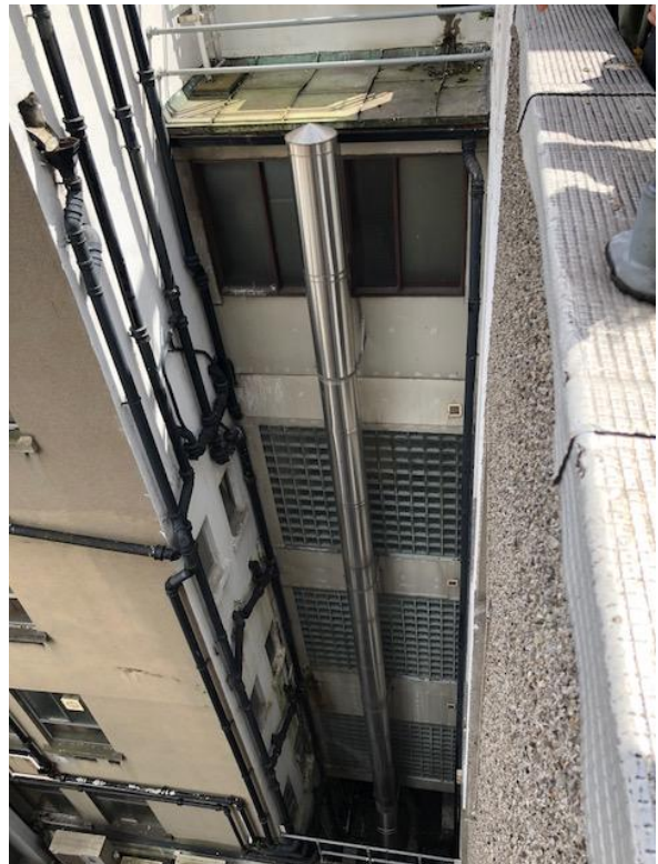
Letter box chute (non-original) that extends the length of the building between Building A and Building B. Link is clad in glass block. The original chute may have been clad in timber.
