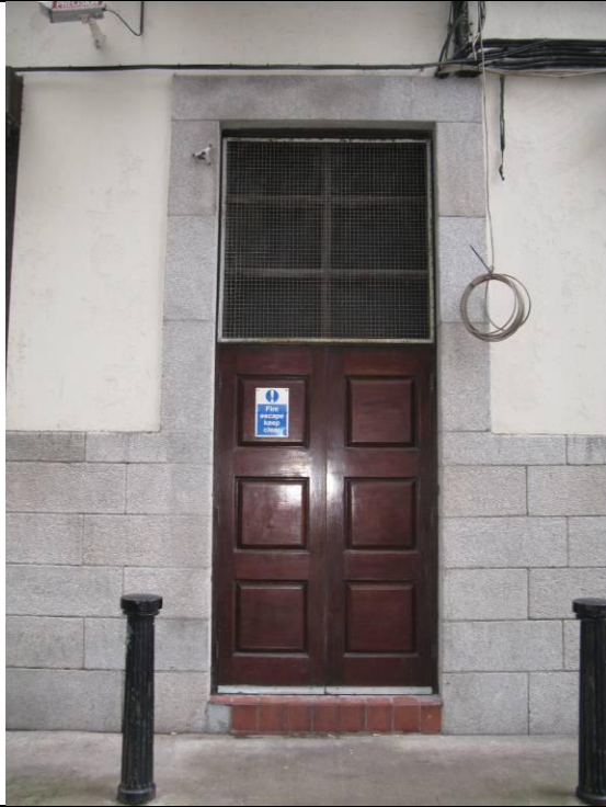
Granite framed, secondary entrance door onto Dawson Lane east elevation
